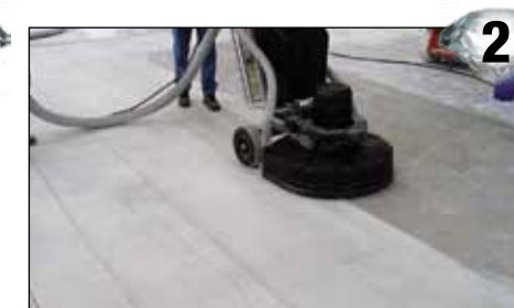
Prep & initial metal-bond diamond grinds
